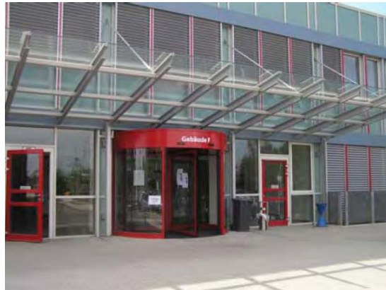
Main Entrance to Building F
